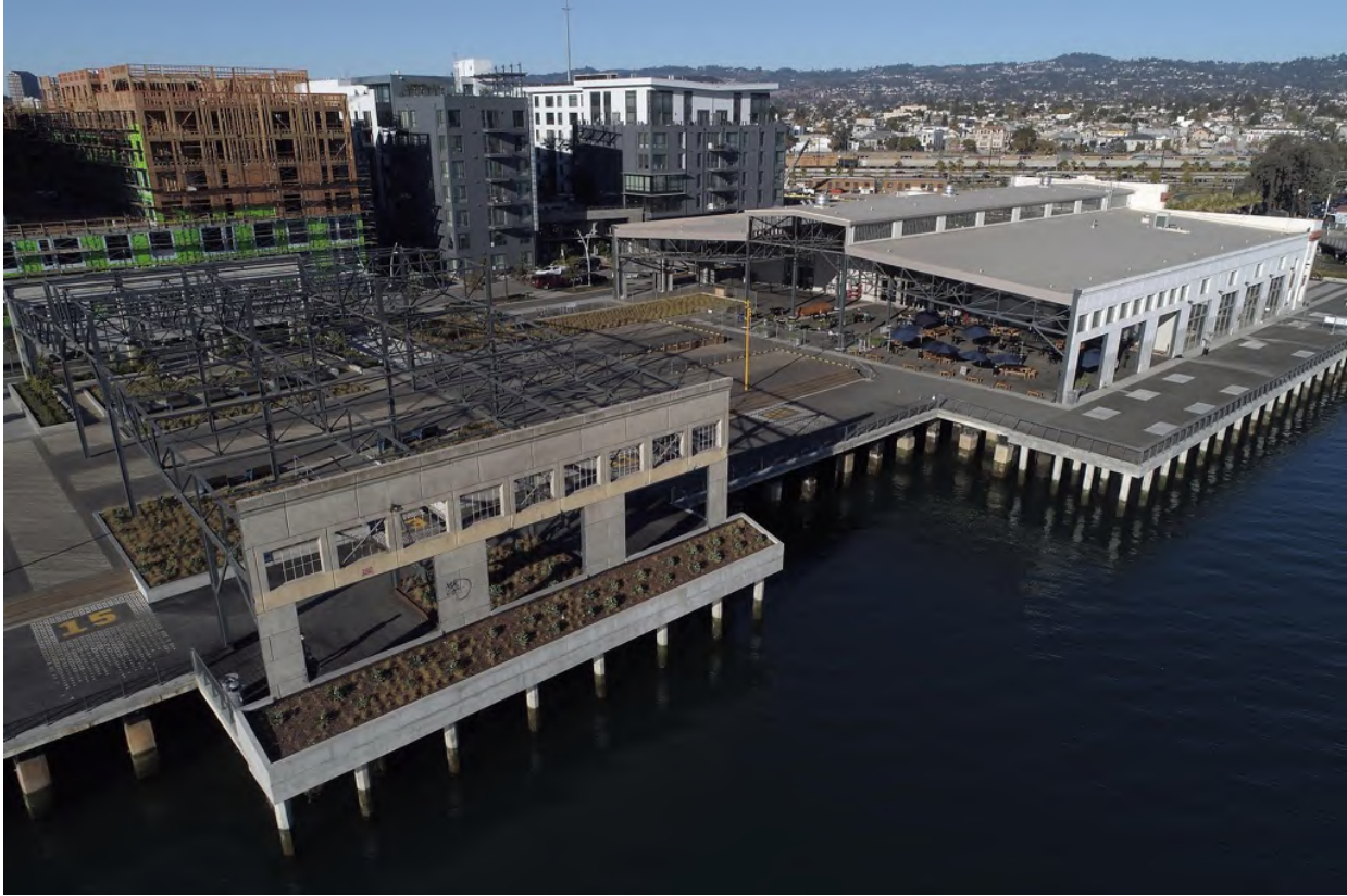
The large back portion of this former cable car barn (later a car dealership) was replaced, and the front section retained and restored.
