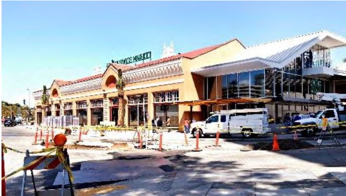
The large back portion of this former cable car barn (later a car dealership) was replaced, and the front section retained and restored.
