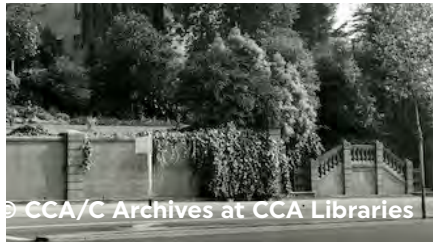
Broadway Wall + Stairs
