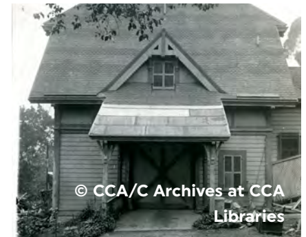
Figure 2.7: Carriage House original opening on east facade
