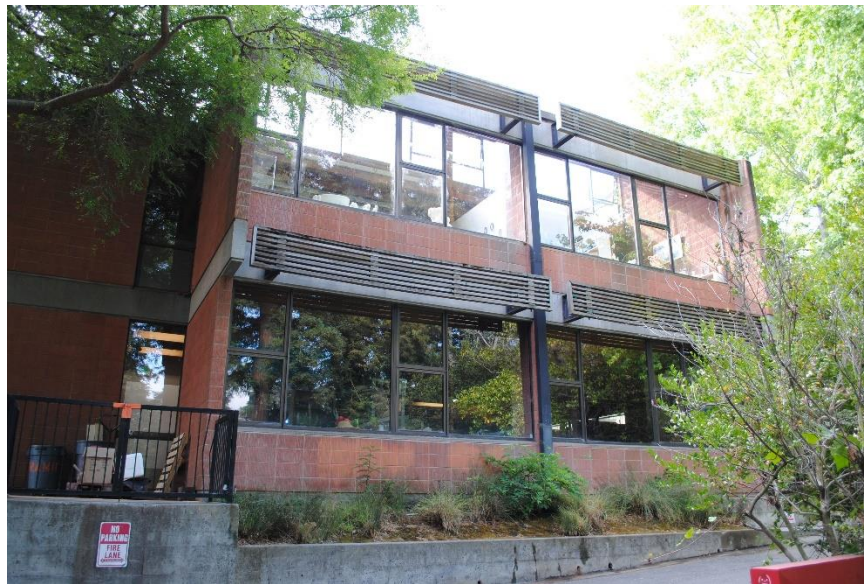
Figure 103. Ceramic Arts Center, south portion of primary (west) façade, facing east.
