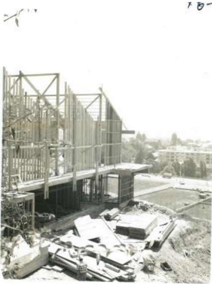
Figure 78. Martinez Hall under construction, 1967-1968. Source: CCA Libraries Special Collections.
