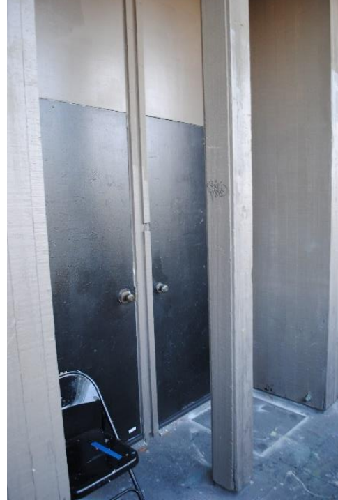
Figure 69. Typical recessed entrance with two tall metal doors, located on the second story primary façade.
