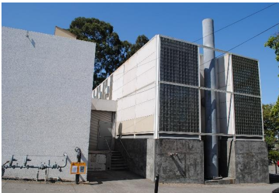
Figure 141. East and north facades of the Barclay Simpson Sculpture Studio, looking southwest. The Shaklee Building (left) is attached by the central hyphen volume.
