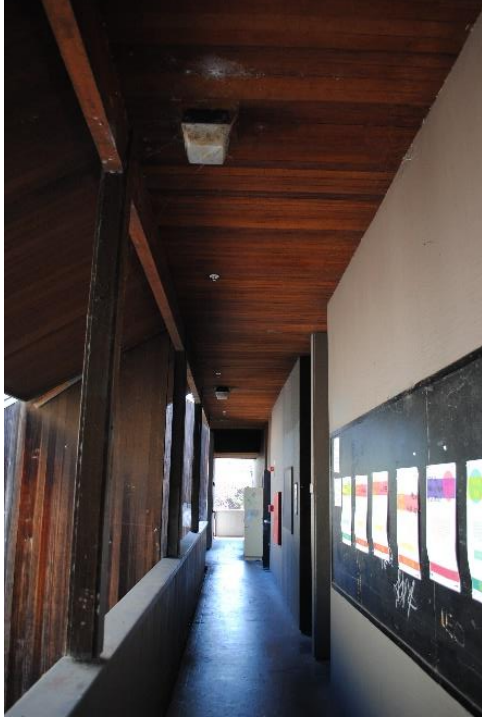
Figure 68. View of exterior hallway along primary façade second story, looking north.
