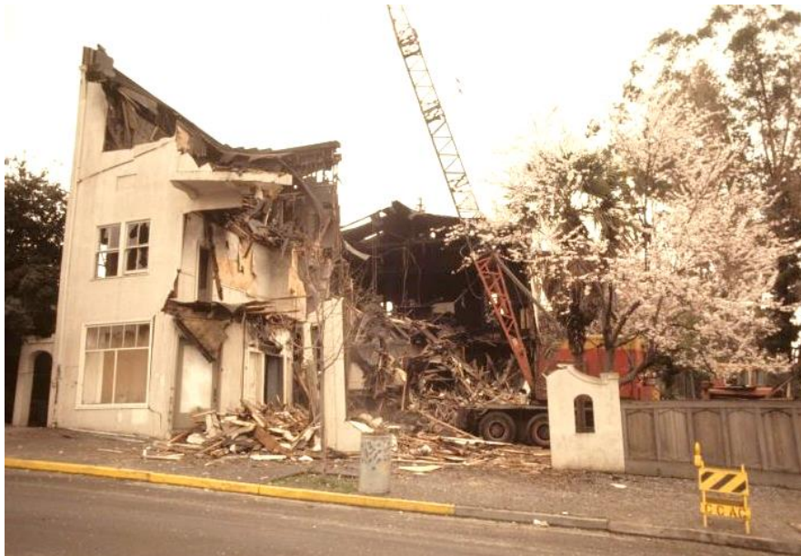
Figure 217. Demolition of Guild Hall after fire in 1971. Source: CCA Libraries Special Collections.
