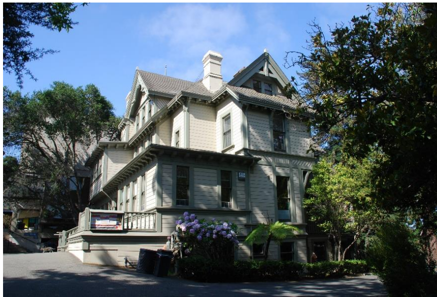
Figure 11. Macky Hall, north façade, partial view, facing southwest.
