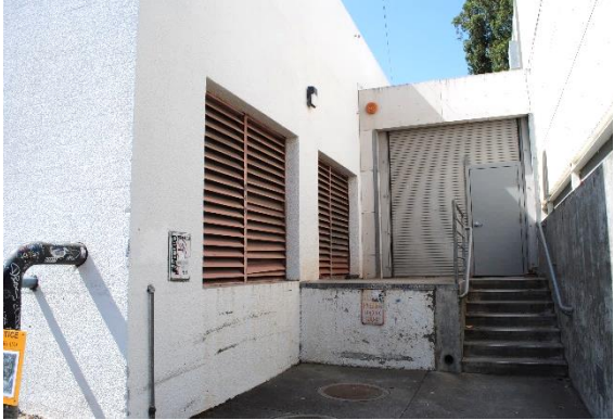
Figure 122. Two large vented openings at the north end of the west façade of Shaklee Building (left), looking south. A hyphen addition attaches to Barclay Simpson Sculpture Studio (right).
