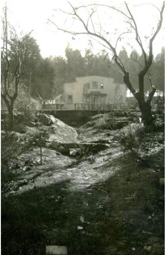
Figure 197. Site and barn, 1926. Source: CCA Libraries Special Collections.
