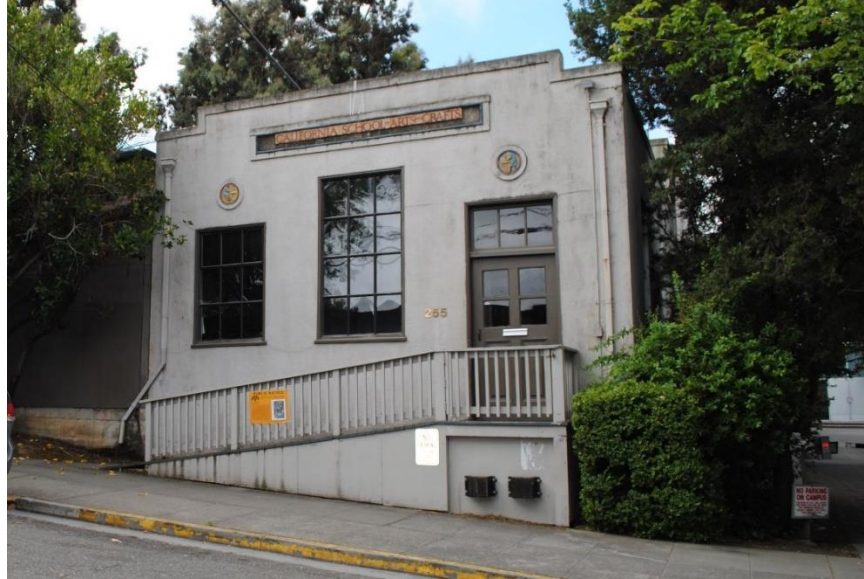
Figure 37. Facilities Building, primary (north) façade, facing south.
