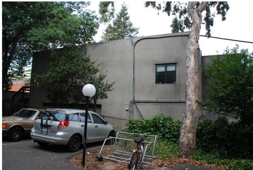
Figure 136. Partial view of the east façade of the Oliver & Ralls Building, facing west.
