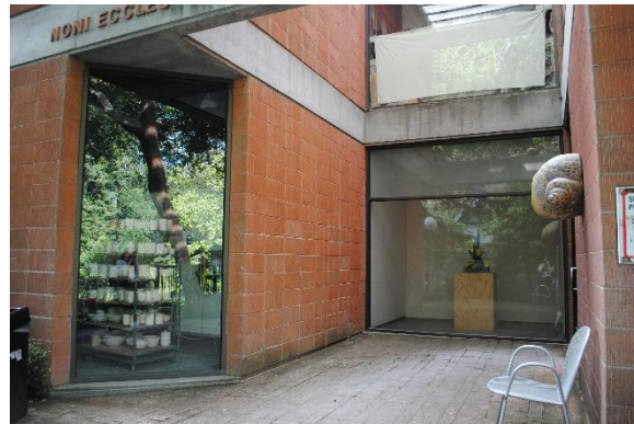
Figure 102. Chamfered corner of the first story of the north volume of the Ceramic Arts Center, featuring a fully glazed window wall with views to the kiln area, looking northeast.
