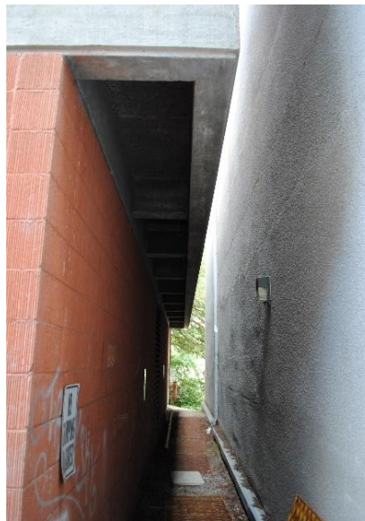
Figure 110. North façade of the Ceramic Arts Center (left), several feet from the Oliver & Ralls Building (right), looking west.
