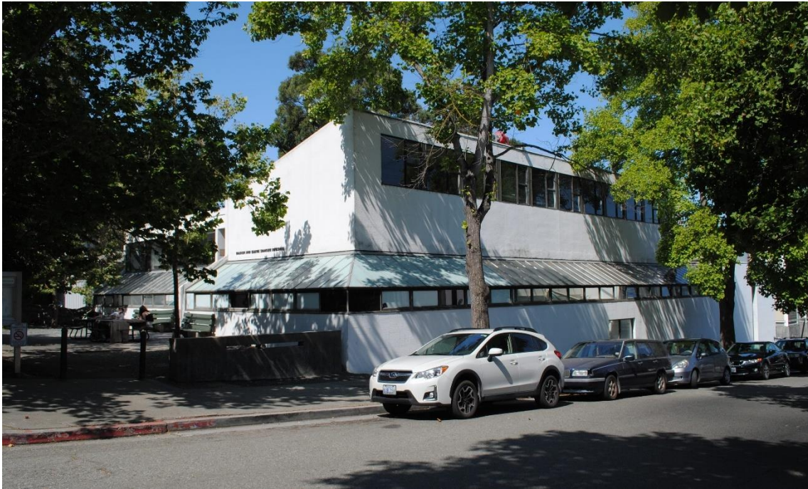
Figure 114. Shaklee Building, oblique view of primary (east) and north facades, looking southwest. North shed roof volume is visible.
