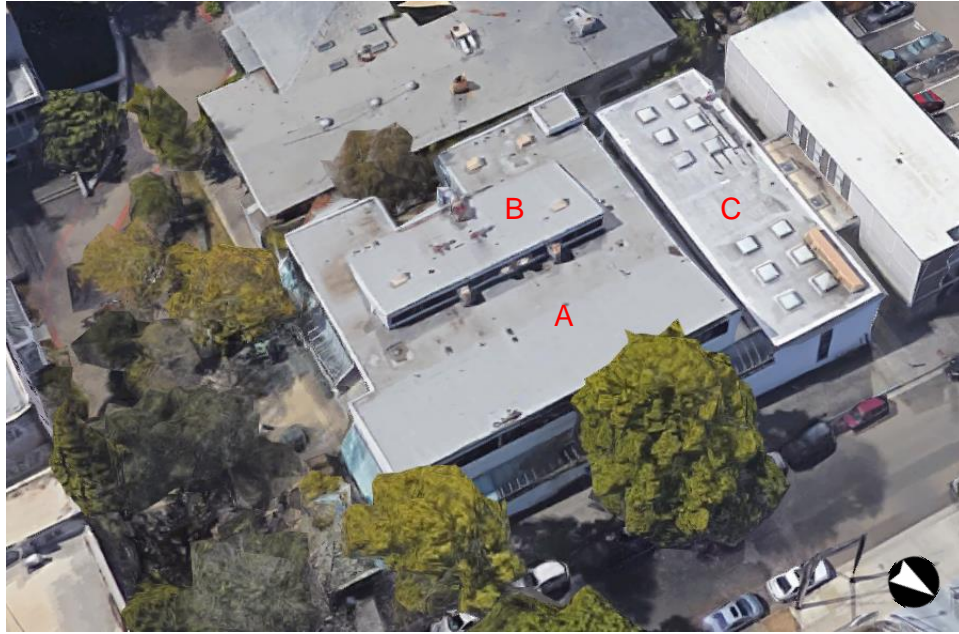
Figure 115. Bird's-eye view of the Shaklee Building. A = north volume with shed roof; B = south volume with flat roof and central shed roof clerestory; C = west volume with flat roof. Source: Google Maps. Edited by Page & Turnbull.
