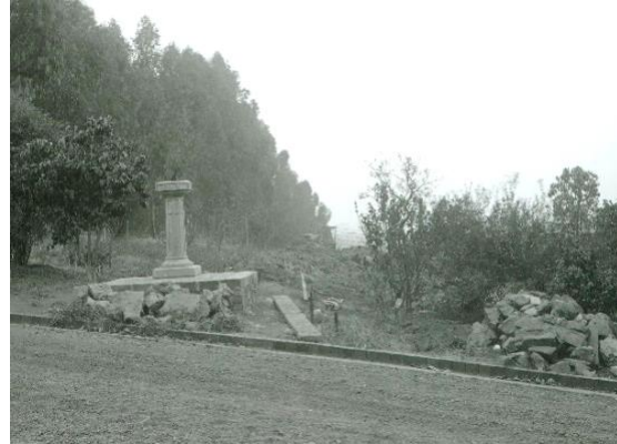
Figure 158. Sundial in southwest corner of campus, September 6, 1929. Source: CCA Libraries Special Collections.
