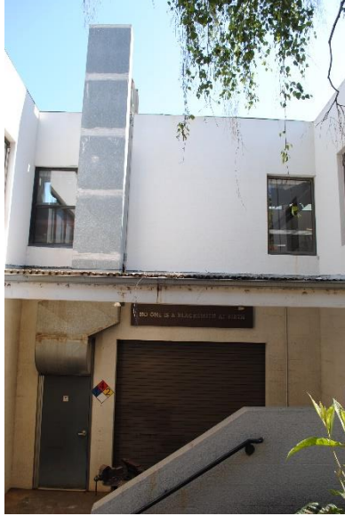
Figure 126. Shaklee Building, two-story recess with entrance on south façade, facing north.
