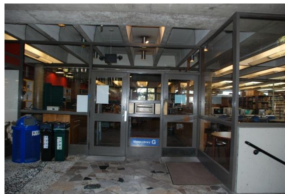
Figure 87. Founders Hall, north façade Meyer Library entrance detail, facing south.
