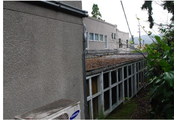
Figure 46: The B Building east façade, facing north.
