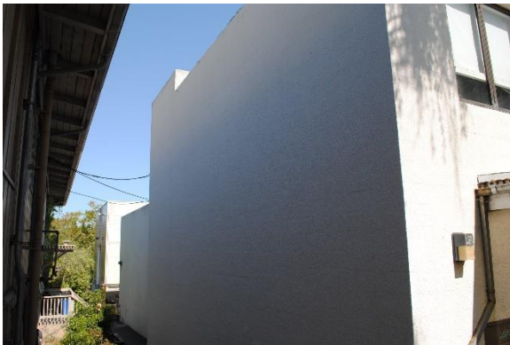
Figure 124. Un-fenestrated west portion of the south façade of the Shaklee Building, looking northwest.
