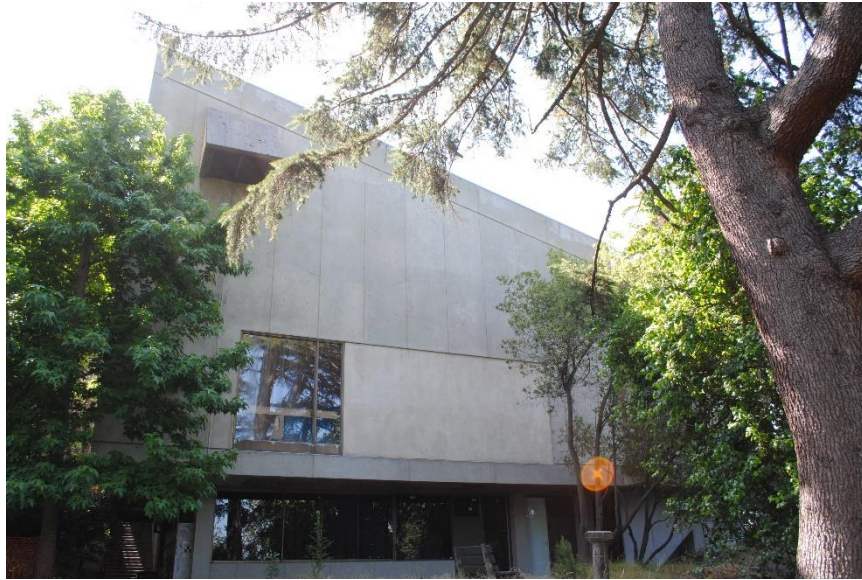
Figure 88. Founders Hall, west façade, facing southeast.
