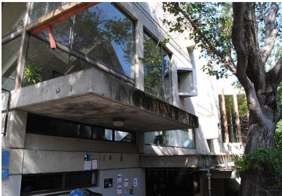
Figure 84. Founders Hall, north façade, facing southwest.
