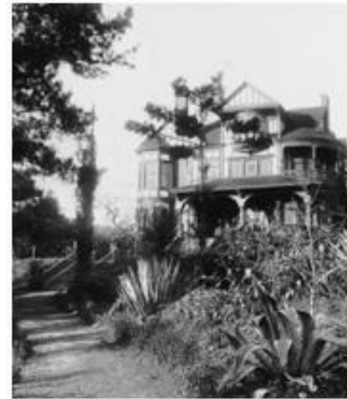
Figure 224. Ella Nichols Park residence, San Rafael, Clinton Day, architect, c. 1888. Source: Falkirke Cultural Center website, http://www.falkirkculturalcenter.org/falkirk-architecture/ .
