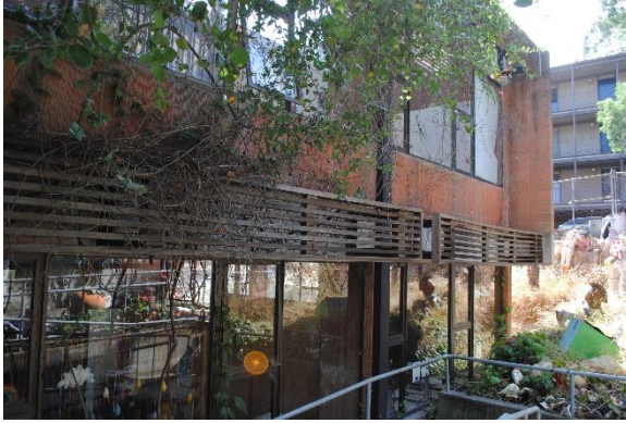
Figure 104. Ceramic Arts Center, portion of south façade with trellis detail, looking northeast.
