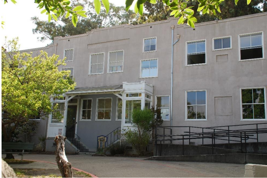
Figure 43. The B Building, west façade, facing northeast.
