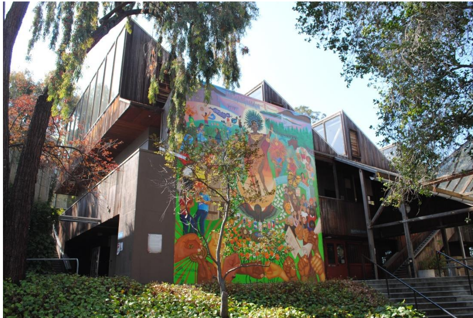
Figure 63. Martinez Hall, west (primary) façade and partial view of north façade, facing southeast.
