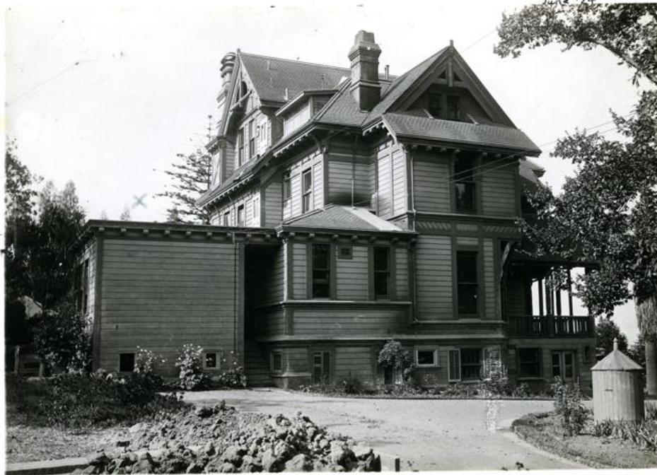
Figure 15. North facade of Macky Hall, June 1924, showing early roof attachment of rear one-story building. Source: CCA Library Special Collections.
