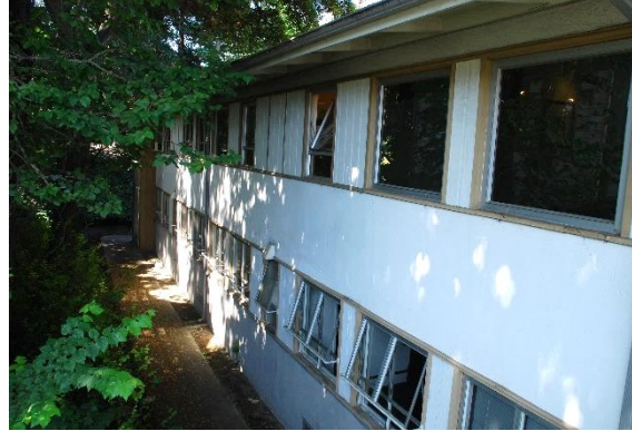
Figure 51. Irwin Student Center, south portion of east façade, partial view, facing southwest.
