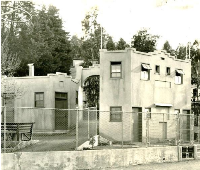
Figure 228. Shower Building, 1930, facing southeast, no longer extant.
