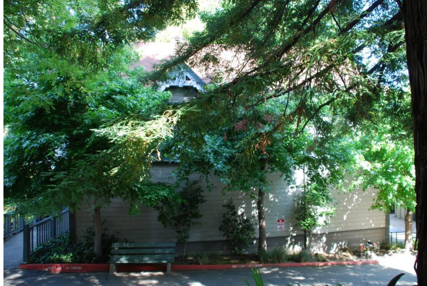
Figure 19. Carriage House, east façade, partial view, facing west.
