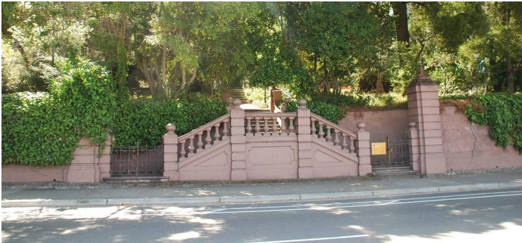
Figure 26. Broadway Wall stairs, west of Macky Hall, looking east.
