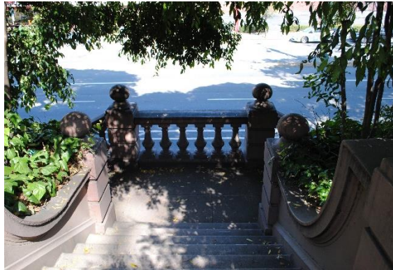
Figure 30. Broadway Wall, upper interior portion of stair, looking west.
