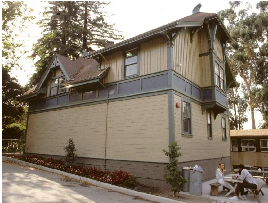
Figure 25. North and east facades of Carriage House shortly after it was placed on its current foundation. Source: CCA Libraries Special Collections.
