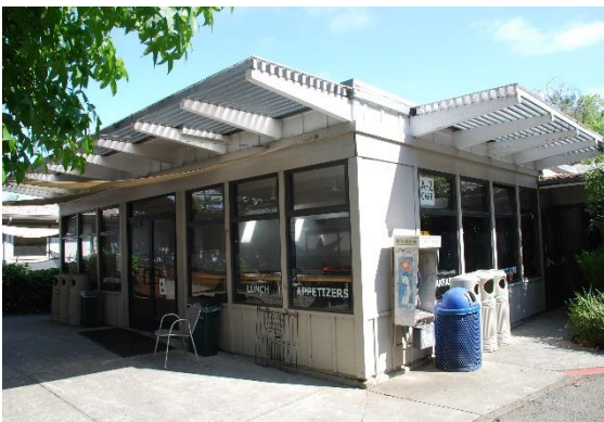
Figure 58. A-2 Cafe, south and east façades, facing northwest.
