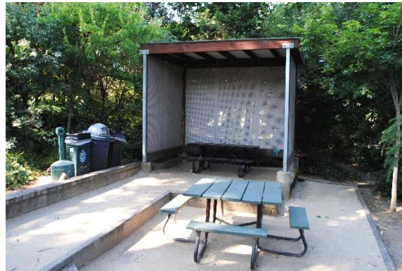
Figure 179. Wood and metal shade structure west of Eucalyptus Row, built at an unknown date.
