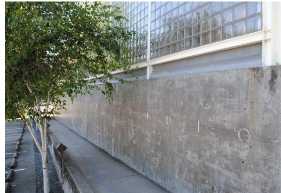
Figure 139. Galvanized metal louvers above the concrete base, within the steel grid frame, looking northeast.
