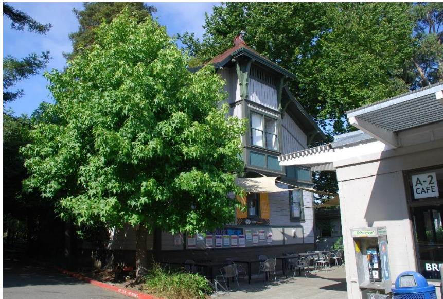
Figure 20. Carriage House, north façade, facing southwest.
