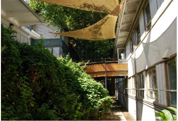
Figure 50. Bridge to the primary entrance of Irwin Student Center on the second floor, looking south.
